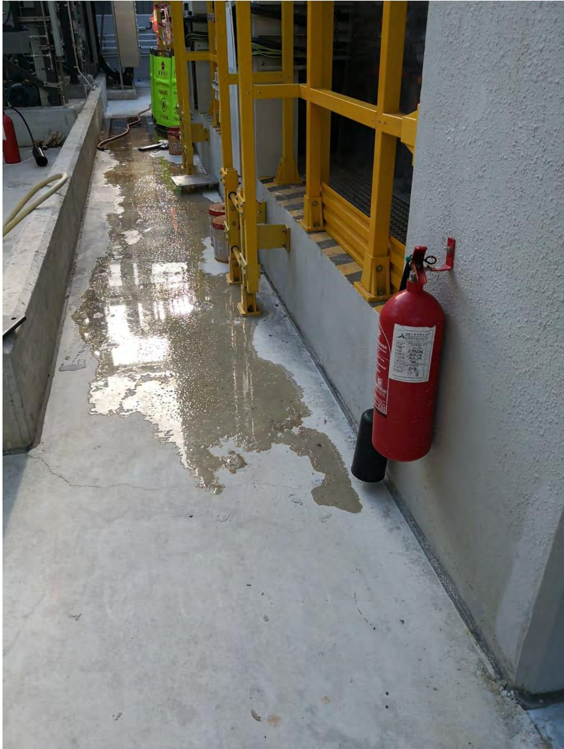
Chemical leakage observed on Building 1 roof.
